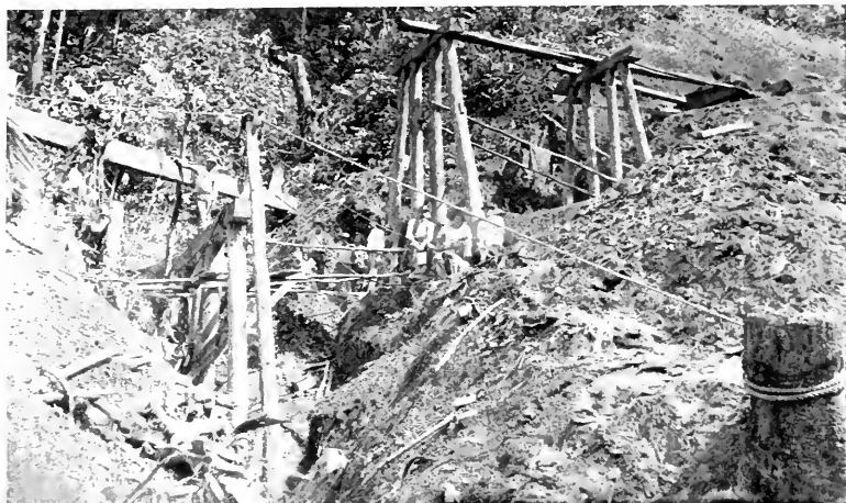
BUILDING A TRESTLE.
